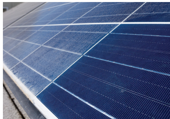
Figure 7. Uniform soiling pattern commonly found on large systems.
